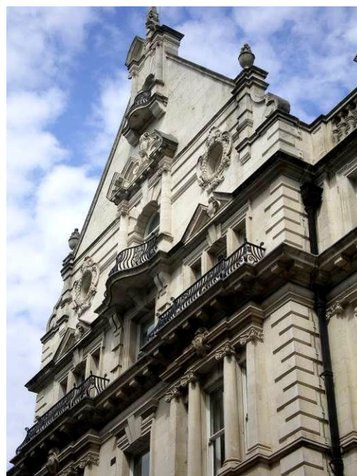
Telephone House (detail)
